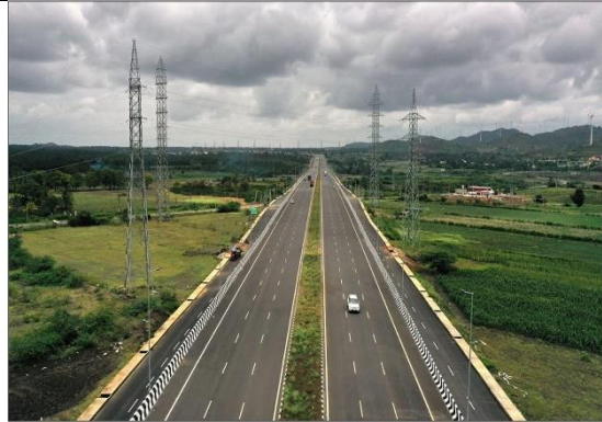
Note: Pic for representation purposes only Nelamangala Tumkur 10 lane Expressway Project cost Rs. 844 crore
